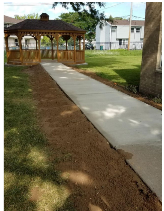
New sidewalk and gazebo at Hudson Ridge Tower
