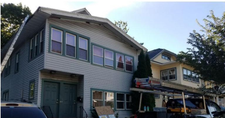
Roof replacements at scattered sites
