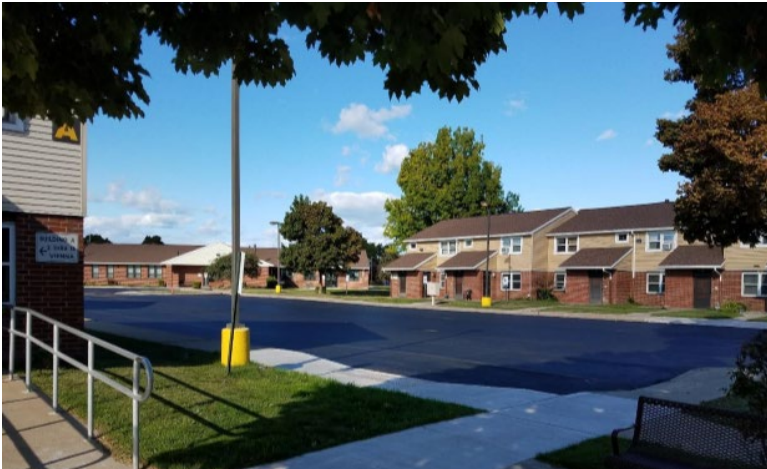
Site improvements at Lena Gantt Estates
