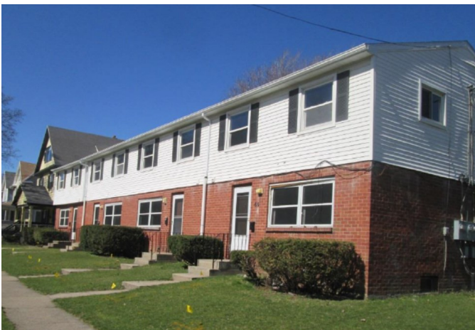
Exterior before rehabilitation
