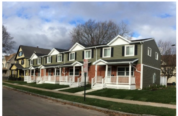
Exterior after rehabilitation
