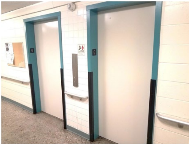
Upgrading elevators at five high rise locations within Danforth Tower West.
